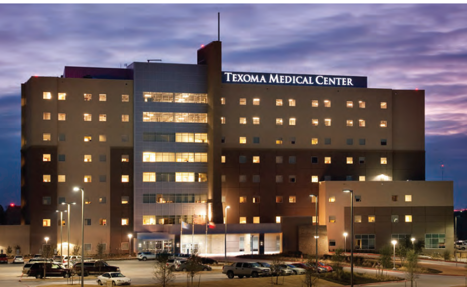
The new Texoma Medical Center, a $130 million replacement hospital, opened in December 2009.
